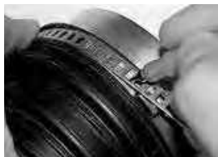
Step 2 Determine the clamp length.
